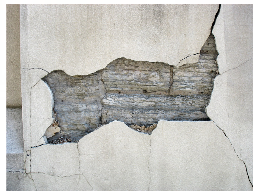
.... not shaky, unstable foundations
